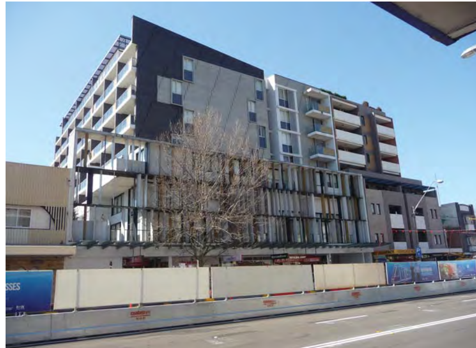
Figure 29: New Mixed Use Development
